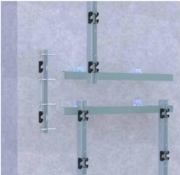
2. Insert the lower set of locating pins of the setting out tool into the top set of holes in the lower modular click rail.
