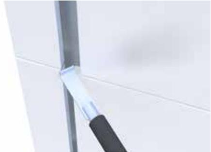
1. To remove an individual panel from the façade, the panel above it must first be unclicked at its lower edge. When using the panel removing tool with round grip, the panel may need to be slid to the one side to create sufficient space to insert the tool into the vertical joint. Insert wedges and unlock the fixed point clamp. Slide the panel to the side and relock the fixed point clamp. Remove the wedges.
